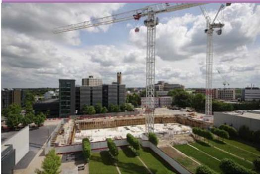
Work is continuing on the site of the new SCI building which is on track for completion in 2018. The basement slab is now complete and preliminary works have started for the concrete frame.
